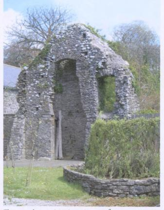
These are the remains of a T-shaped 14<sup>th</sup> century Hall House, surviving only as a full height cross wall with fireplace, foundations and first floor doorway. The ground floor would probably have been the kitchen area with the living space on the first floor. Go S on the "new road" built when the original road was closed (see Walk 2)
