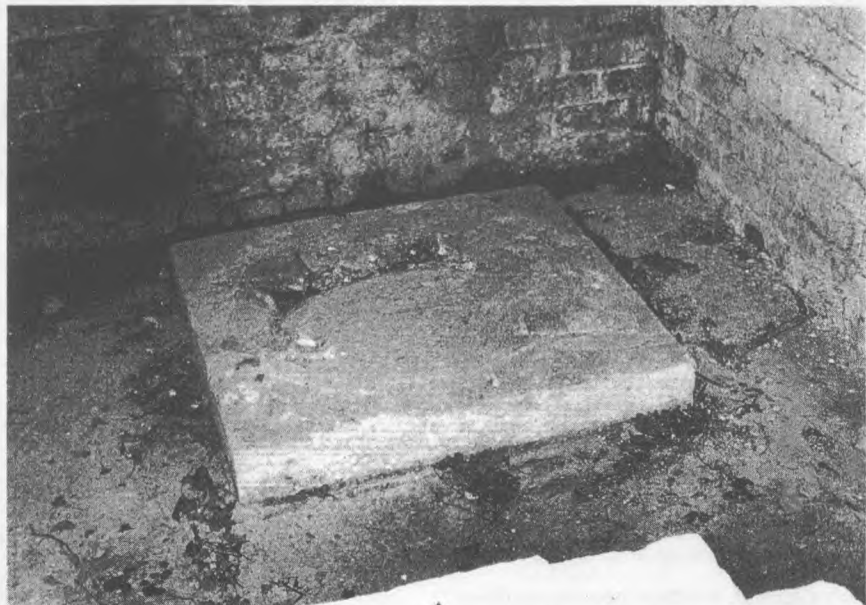
The remains of the trap door to the first ill-fated tunnel. The subsidence of the base of the stove platform might have been caused by the stove having been placed on fresh soft concrete soon after the trap door was sealed after discovery. A PoW had scribbled on the walls of the hut 'to the tunnel' with an arrow pointing in the wrong direction, no doubt to taunt the guards after the discovery. The precise location of this tunnel is not known.
