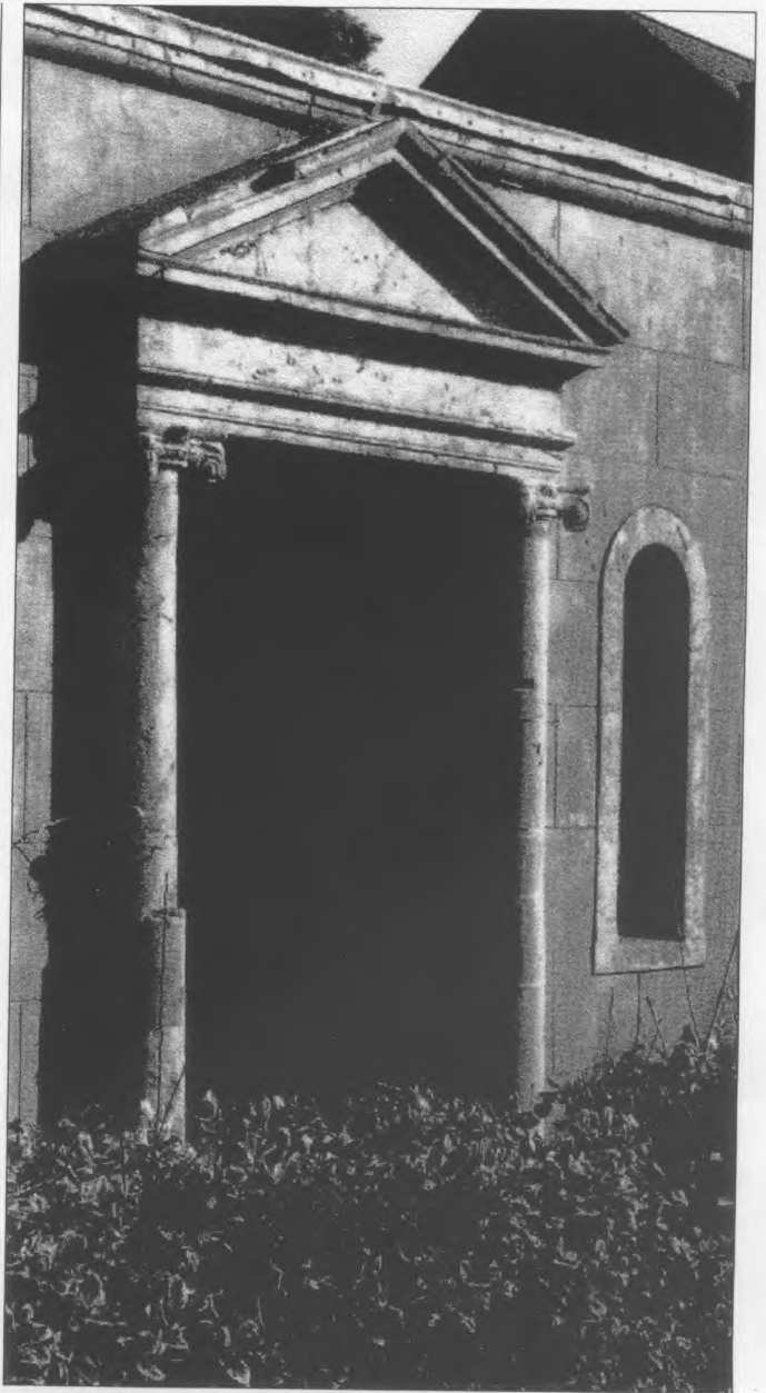
Fig.3 The classical pedimented stone doorway in the back wall of the house.
