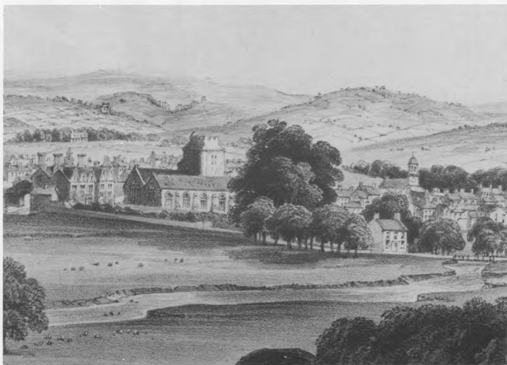
Holy Cross Church from the south, with the former Grammar School left and Town Hall right
