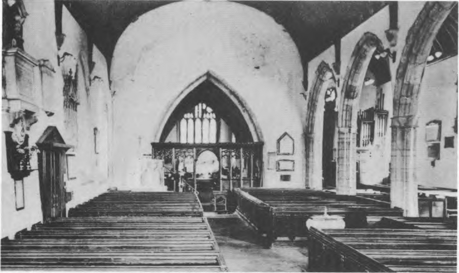
The nave before the removal of the screen
