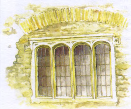
Mullioned window with arch headed lights.
