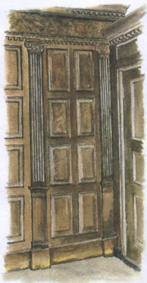
Oak panelling with fluted pilasters.
