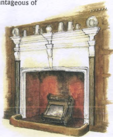
Classical dressed stone fireplace.
