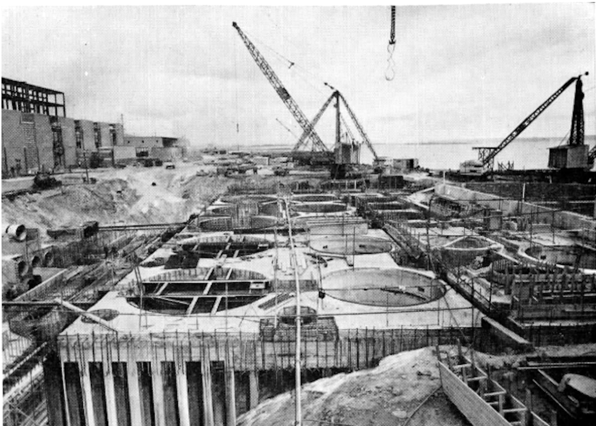
CIRCULATING WATER PUMP HOUSE UNDER CONSTRUCTION
