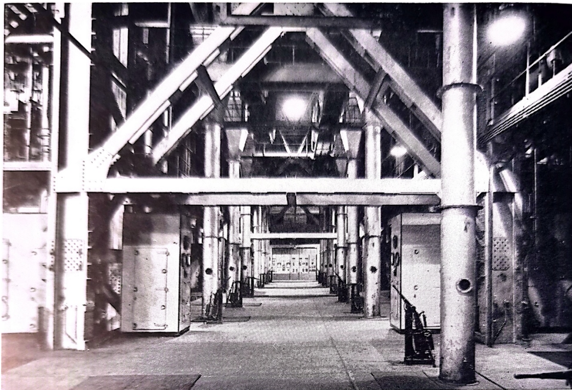
BOILER HOUSE AISLE
