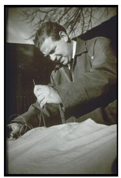
Over the centuries hide was replaced by calico. The cloth is stitched in place and then painted with a sealant to make iut hard and waterproof. The woven gunwhale is sometimes replaced with sawn ash. Today some coracles are made from fibreclase
