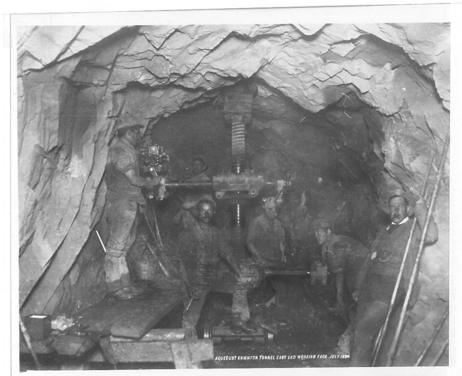
Elan Valley Aqueduct. Knighton Tunnel workings.
