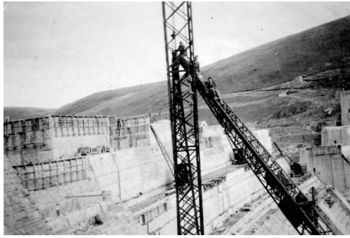
Black and white photograph of the construction of Claerwen Dam.
